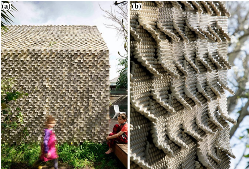
Fig. 12 3D printed ceramic tiles on façade. (Color figure online)
