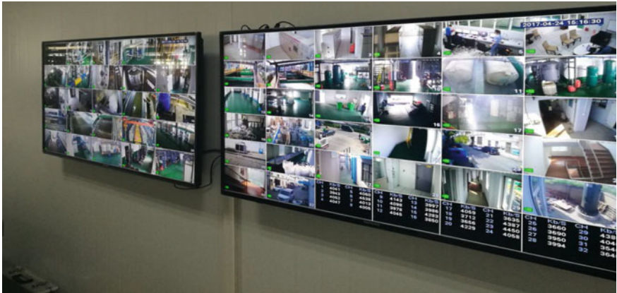
Fig. 5 PLC control system of Futianbao SCR “zero emission system”. (Color figure online)
