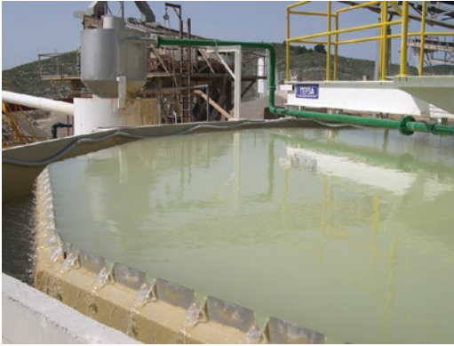
■ Fig. 2.29 Nonmechanical sedimentation classifier. (Image courtesy of TEFSA)
