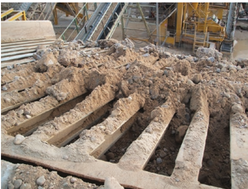
■ Fig. 2.31 Grizzly screen used to remove large boulders
