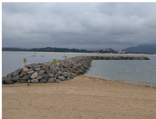
■ Fig. 2.51 Aggregate used as armourstone (Santander, Spain)
