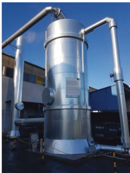
Fig. 17.7 Full-scale CTBB and control panel of its automation system. (Ekoinwentyka Ltd.)
