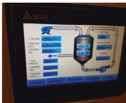
Fig. 17.7 Full-scale CTBB and control panel of its automation system. (Ekoinwentyka Ltd.)
