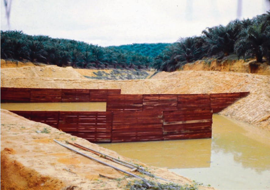
Fig. 14 Anaerobic and facultative ponds to break down palm oil effluent in Pahang, Malaysia (1975)
