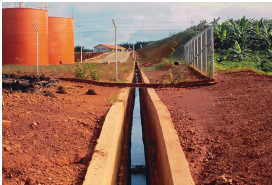
Fig. 10 An effluent discharge canal at a palm oil mill in Pahang, Malaysia (1974)
