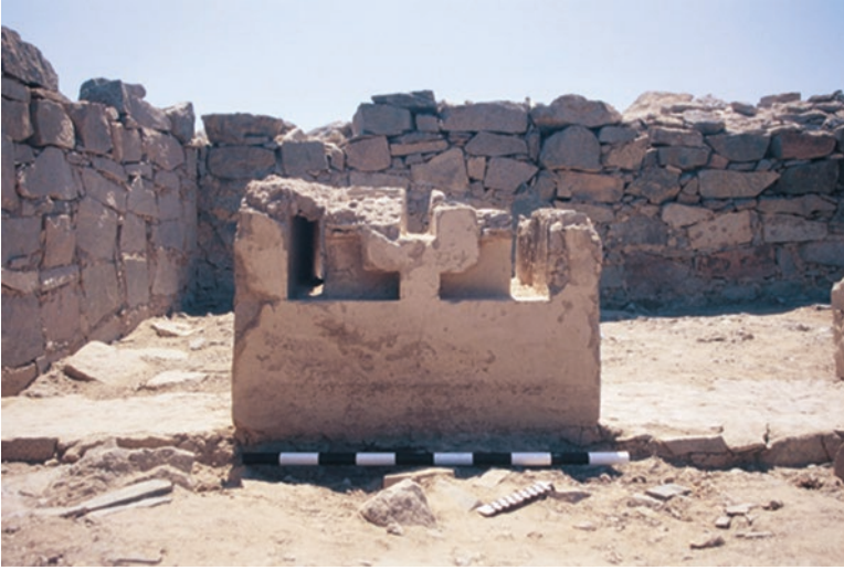
Fig. 7 Slitted pillar preserved in Room 3, Temple of the Pillars. The foundation can be seen under the pillar
