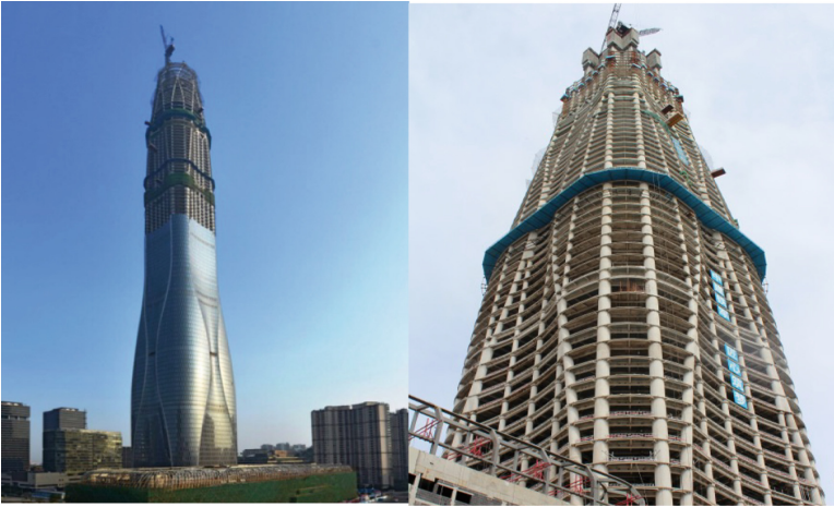
Fig. 2. Project under construction (Source: skyscrapercenter)
