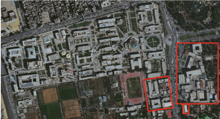
Fig. 1. Worldview-3 image of Cairo University campus with Faculty of Engineering campus in red frames.
