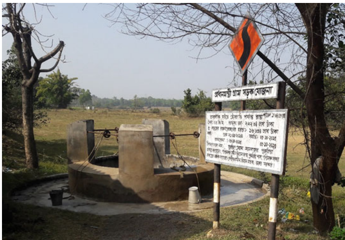
Fig. 23.6 A typical dug well in Purulia district
