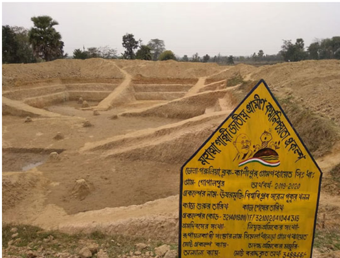
Fig. 23.4 Excavation of a pond in Kashipur gram panchayat in Purulia district
