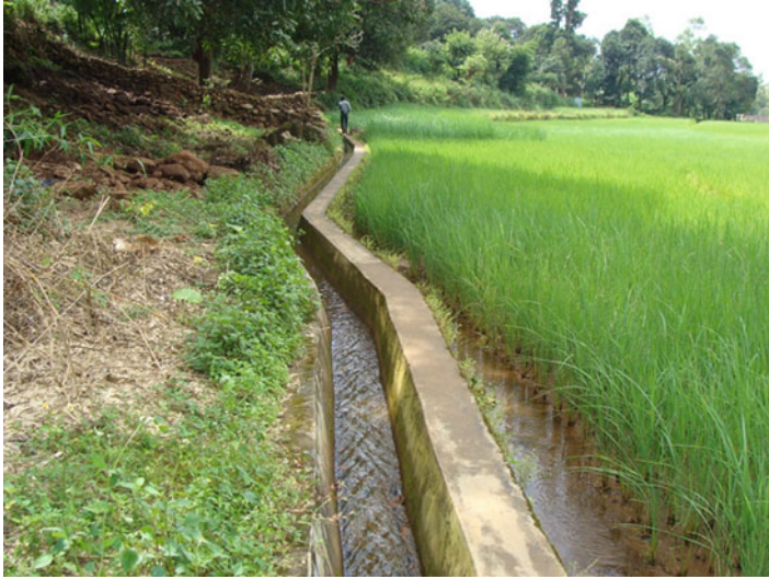
Fig. 17.8 Water convey channel to irrigate paddy and vegetable crops in the watershed
