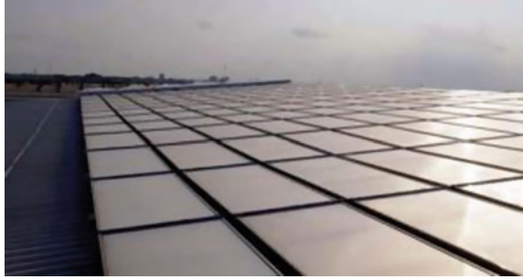
Fig. 11 Solar thermal system for hot air at textile manufacturing plant in Vietnam (Source SHIP [52])
