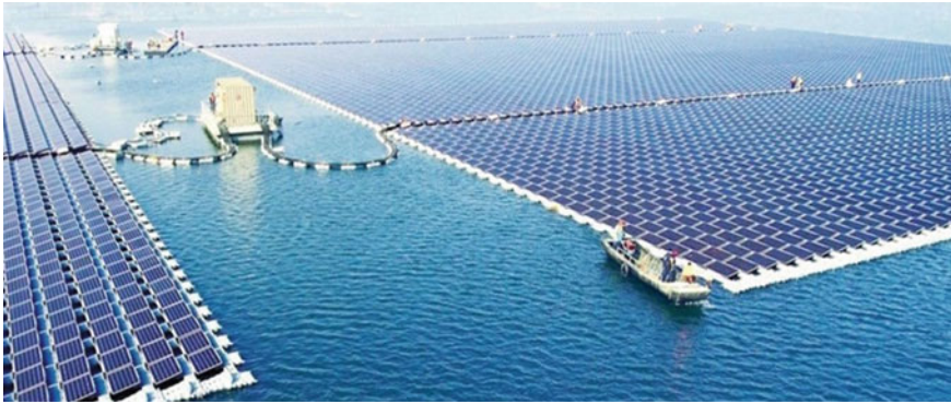
Fig. 2 World’s largest 40 MW floating solar power plant at Huainan, China (Source Brandon [13])
