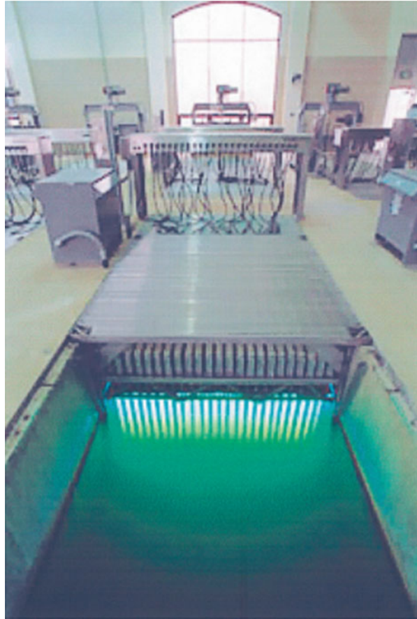
Fig. 6.3 UV treatment for drinking water ( https://www.gigahertz-optik.de/en-us/basics-light-measurement/apps/uv-disinfection-lamp-control/ )
