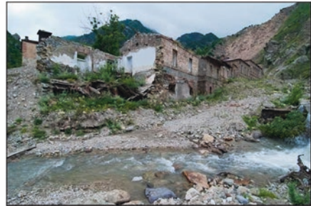
Residential mining houses destroyed by a mudflow.
