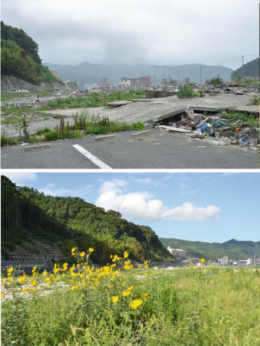
Fig. 25.1 Landscapes in Onagawa city (Miyagi, Japan). This place was destroyed by the tsunami tidal waves reaching 30 meters height on March 11, 2011. The pictures photographed from the same site on Aug 2011 show the serious breakage of buildings and roads (upper, Aug 2) as well as the effective growth of plants (lower, Aug 27). Courtesy, Otoshiro Hiratsuka
