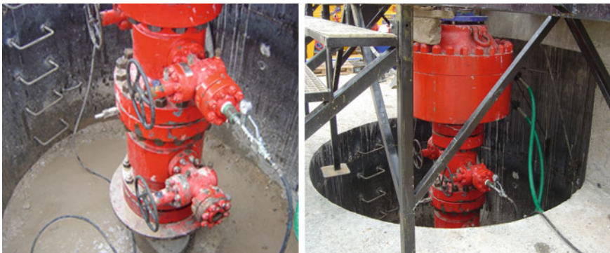
Fig. 6 Installation of BOP and spools during HI well drilling (Courtesy of CIUDEN)
