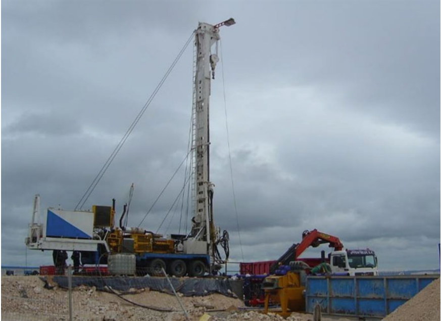
Fig. 3 Rig SEGOQUI 2000 drilling at Hontomín TDP (Courtesy of CIUDEN)
