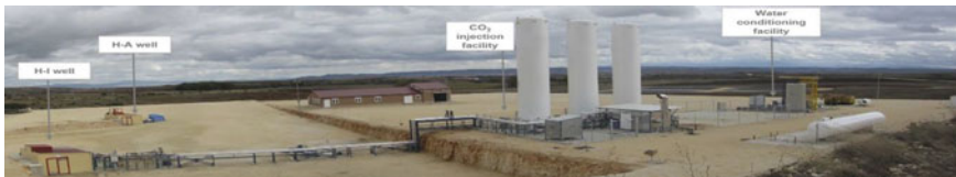
Fig. 7 Panoramic view of Hontomín Technology Development Plant
