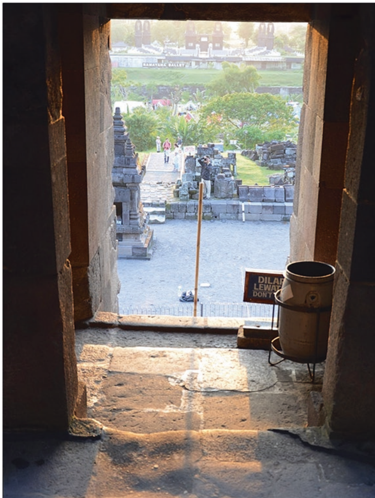
Fig. 14.2 A wooden bar as a sundial placed in the middle of the western chamber entrance of Śiva temple to verify the orientation of the temple.
