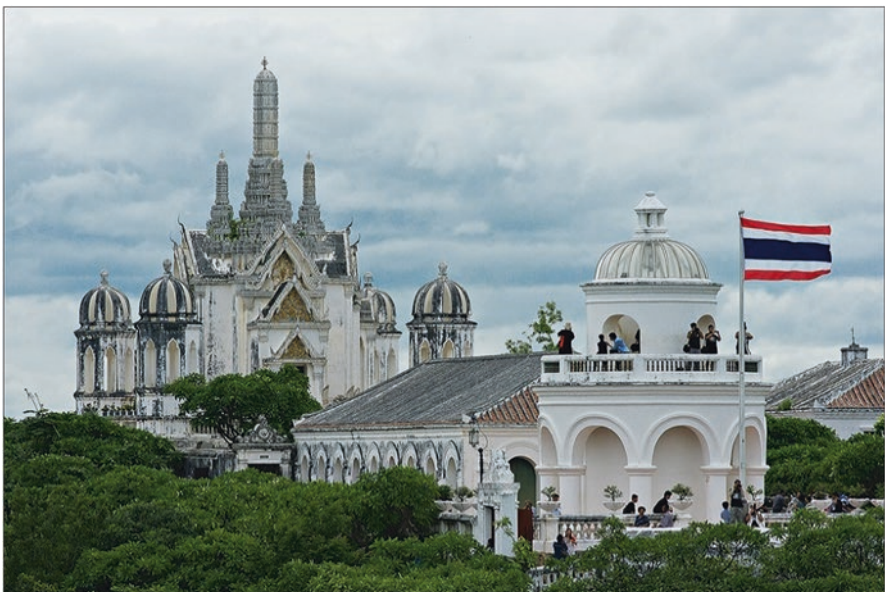
Fig. 6.20 A view of Chatchawan Wiang Chai Hall at Kao Wang showing the recently-restored lighthouse ( https://www.thailandtourismdirectory.go.th/en/info/attraction/detail/itemid/4383 ).
