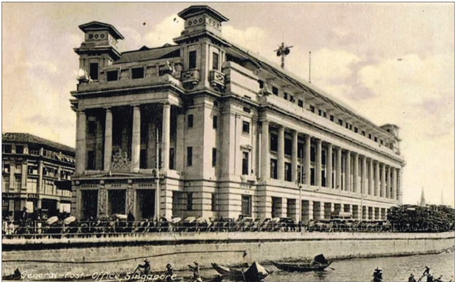
Fig. 12.16 1933 View of Singapore GPO, showing the time discs in their collapsed position (courtesy: Klaus Hülse Collection).
