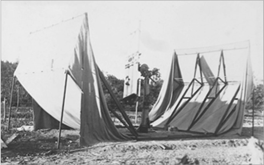
Fig. 10.9 The astrograph safely installed in its ‘observatory’ (photograph: King Prajadhipok Museum).
