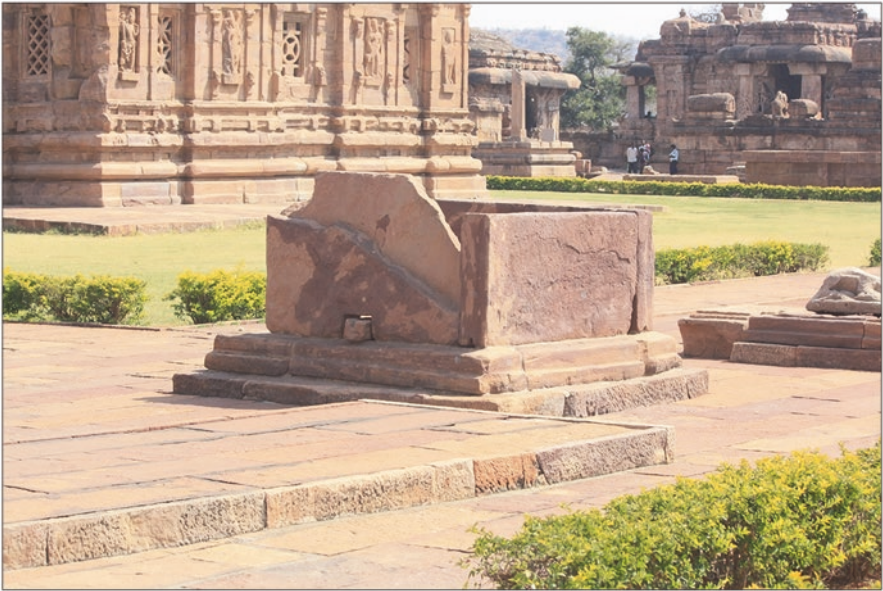
Fig. 21.14 A small shrine at the Pattadakal group of temples in Karnataka, a World Heritage Site, which is constructed in a similar manner as a dolmen. The bigger temples of the site can be seen in the background.
