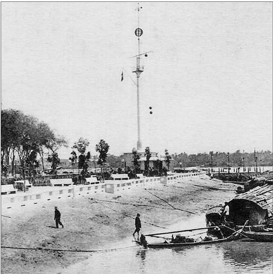
Fig. 12.22 Saigon signal mast and time ball from the river side (Kinns Collection).
