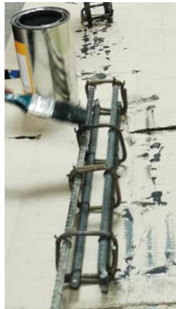
Fig. 3. Applying zinc coating to steel reinforcement cages
