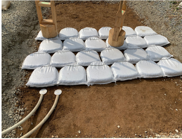
Photo 3. Installation of earth pressure gauges
