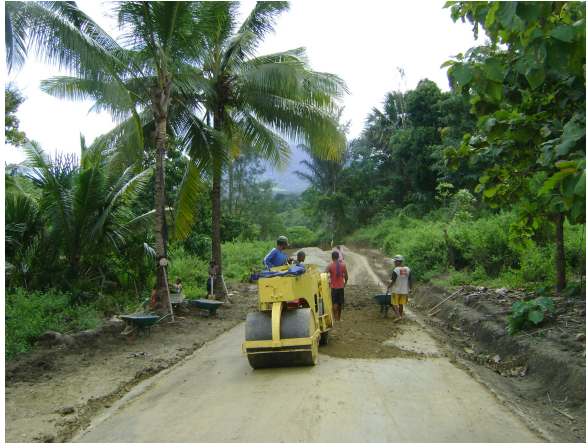
Photo 1. Construction of gravel road with LBT, compaction with equipment
