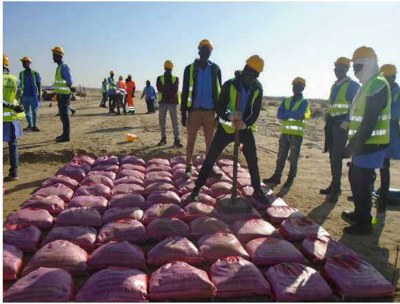
Photo 2. Construction of base course with Do-nou method
