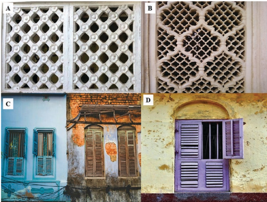
Fig. 7.2 (A, B) Zafris/wall ventilators; (C) window along with the wall ventilators and (D) wall size windows
