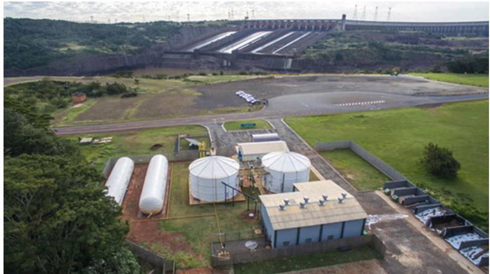
Fig. 3 Aerial view of the demonstration unit—DU ITAIPU
