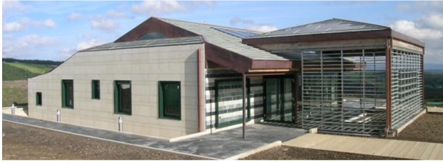
Fig. 1. Sotavento bioclimatic house
