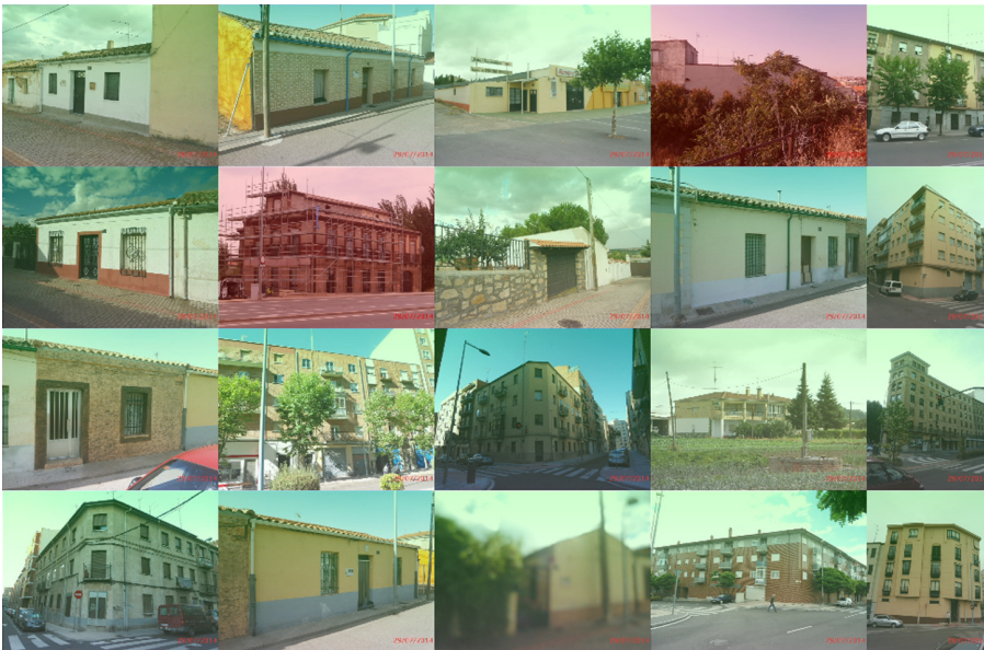
Fig. 2. Obtained results for building classification. Images in red show errors in classification, images in green show successful cases. (Color figure online)
