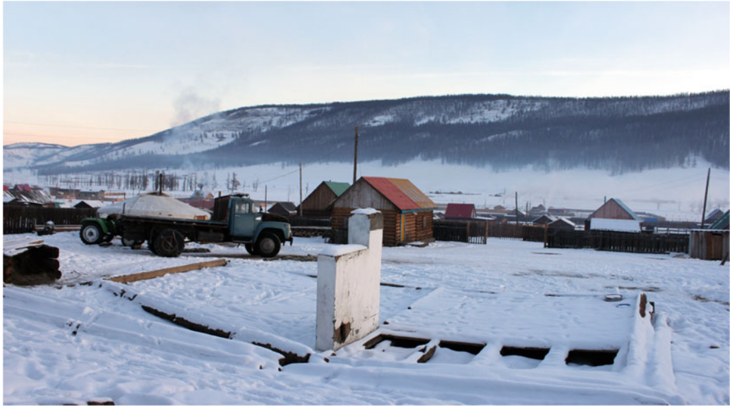
Fig. 7.11 Result of permafrost thawing under the wooden house in Chandmani-Undur sum in north part of Mongolia (photo by A. Dashsteren)
