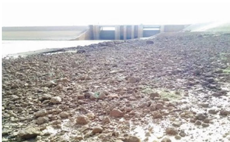
Plate 4 Sand Dome presence in Goronyo Dam
