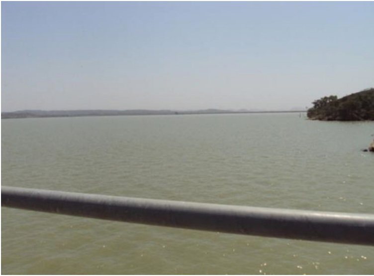
Plate 1 Section of Goronyo Dam from the northern side before 2017
