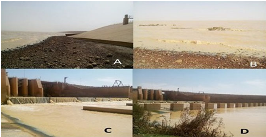
Plate 2 Goronyo Dam Showing Upstream (A–B) and Downstream (C–D)
