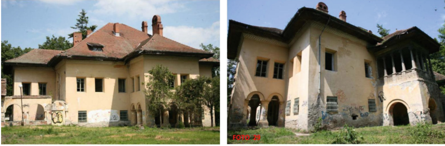
Fig. 5. Main façade of Cantacuzino manor
