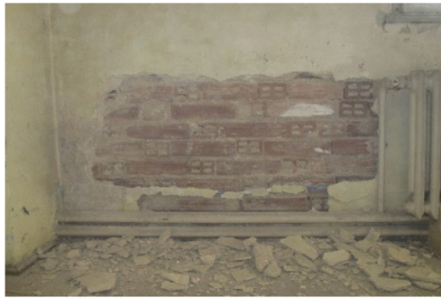
Fig. 7. Plaster exfoliation revealing the non-homogeneity of the masonry walls [16]
