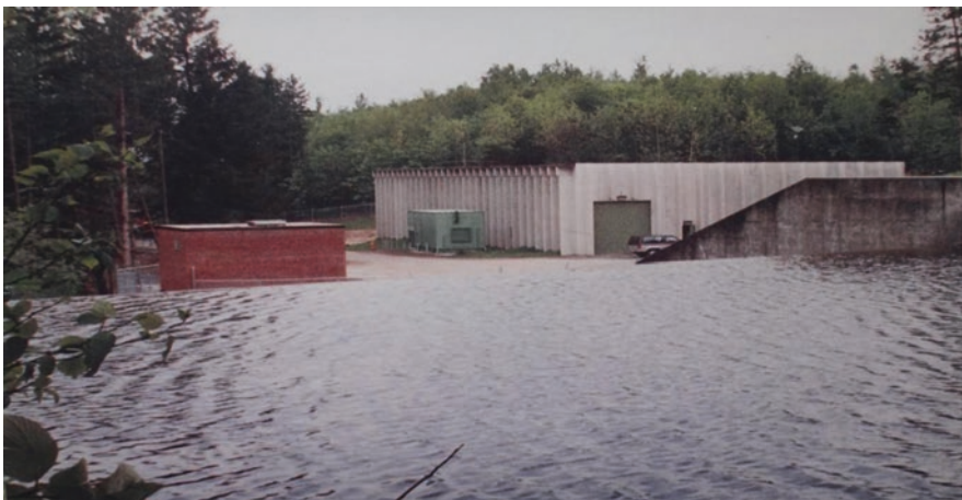
Fig. 8.4 Pittsfield WTP's water treatment buildings are next to the raw water reservoir
