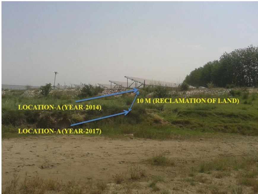
Fig. 6 Huge Siltation and formation of new bank at location-A (in front of power plant) in the year, 2017. Site condition of location-A in the year, 2017 can be compared with the condition in year, 2014 (Fig. 5)
