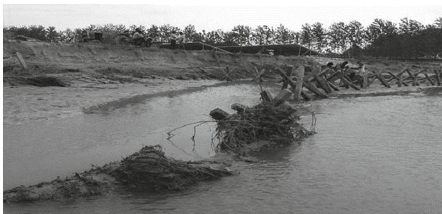
Fig. 8 Trapping of small trees and debris by jetty-field in Solani River, India
