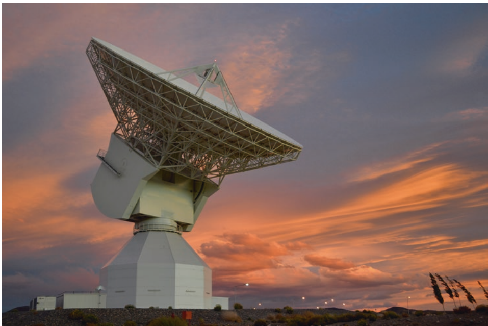
Fig. 5.9: The 35 meter diameter antenna at New Norcia, near Perth, in Western Australia. It was specially built for ESA to ensure reliable communications for deep space missions such as Rosetta. (ESA)
