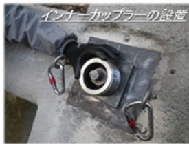
Installation of Inner Coupler
