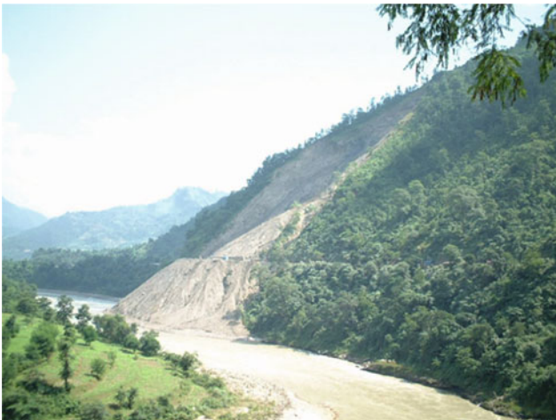
Fig. 13 Picture of slope failure along the Krishanabhi-Kurintar sector of the Prithvi Highway in Nepal (Source Bhattarai et al. 2004)
