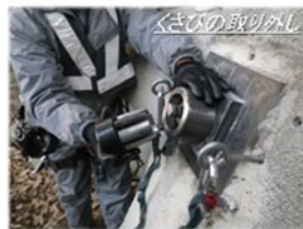
Removal of Wedge
