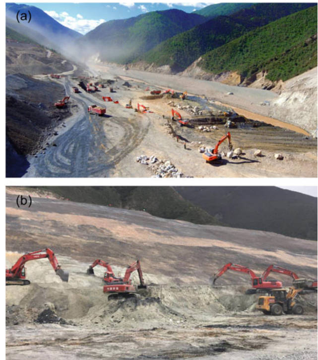
Fig. 15 Actions to prevent the formation of a very large future landslide dam: a removal of the barrier material above 2915 m to make room for future landslide debris; b load removal at the slope crest at Baige (photo credit a SASAC; b Mr. Q. T. Yang)
