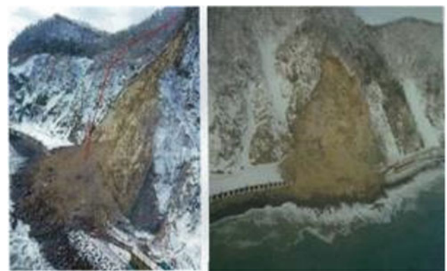
Fig. 10 Bedrock collapse of Shono, Erimo-cho in 2004
