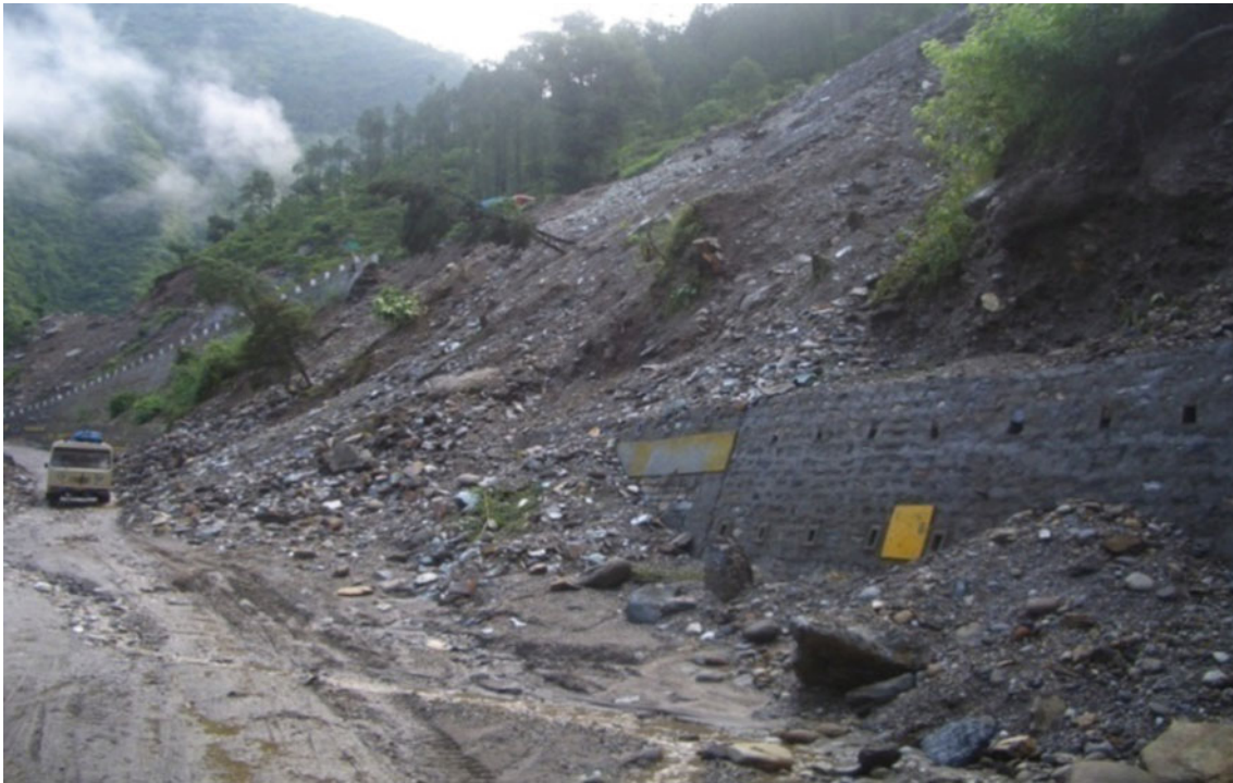
Fig. 1 Completely unstable debris slide due to road excavation in the Lesser Himalayas
