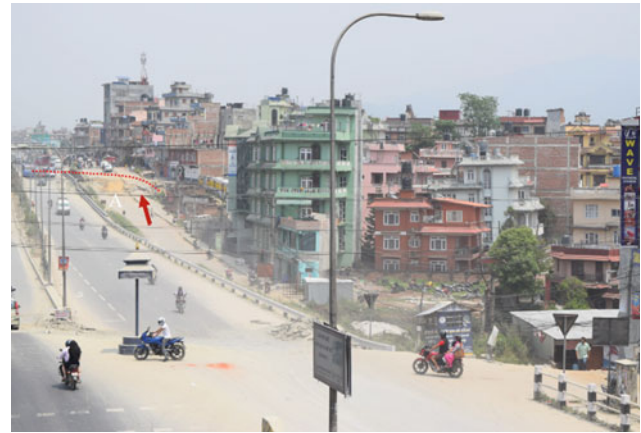
Fig. 6 Seismically induced ground failure site at Lokanthali, Kathmandu after the 2015 Gorkha Earthquake, Nepal
