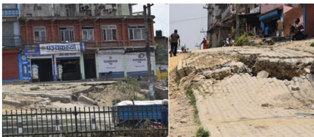
Fig. 19 Pictures of the scarp-like features observed at Lokanthali, Nepal (Source Tiwari et al. 2018)
