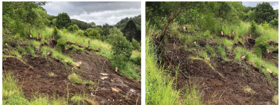
Fig. 9 View of the landslide area (20/Feb/2018)
