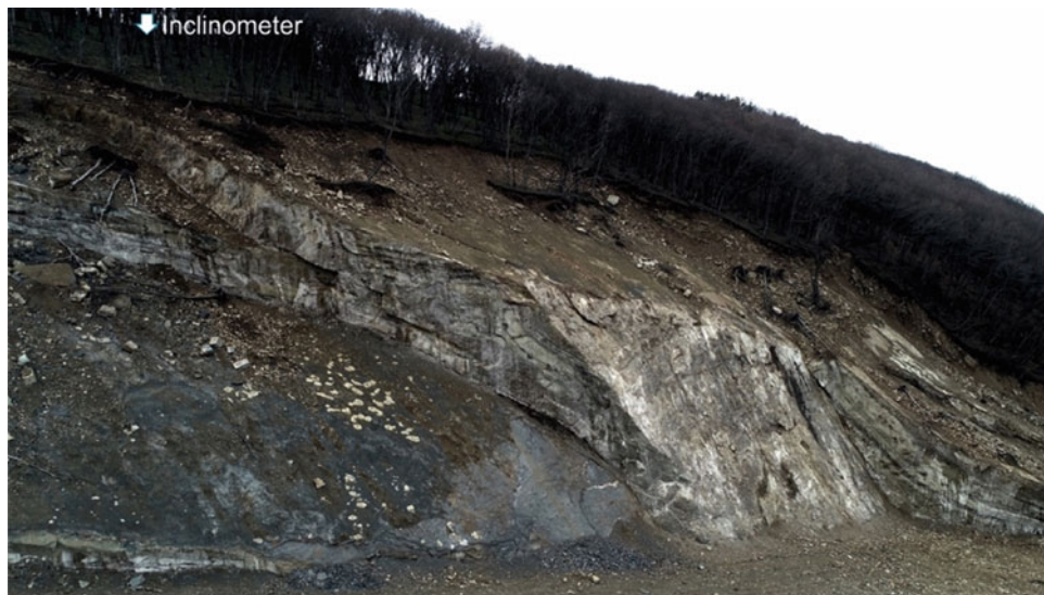
Fig. 3 Large cliff in the upper part of the landslide that is being monitored with an inclinometer
