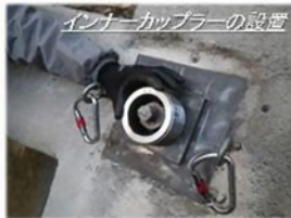
Installation of Inner Coupler
