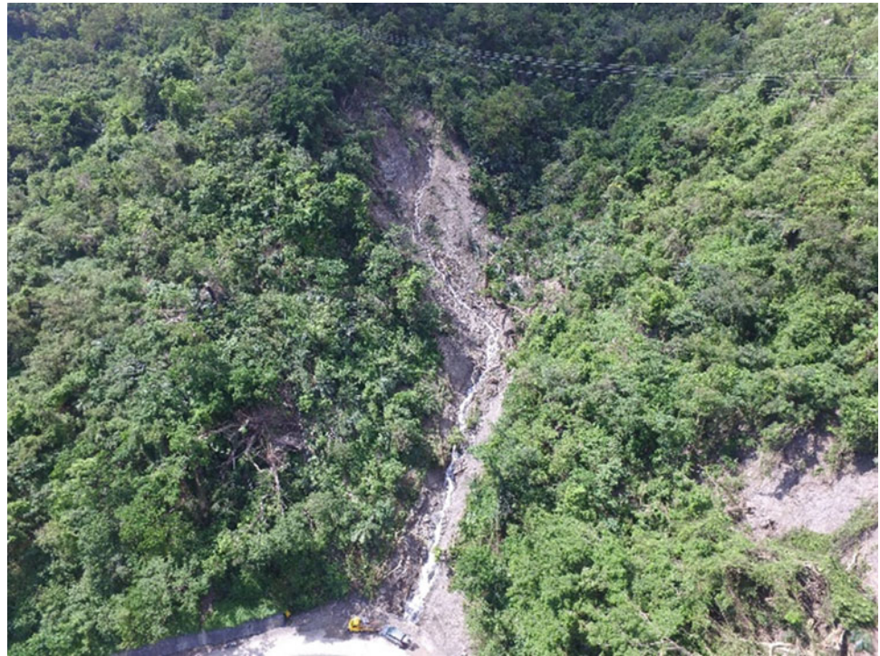
Fig. 7 Photo of route 9 410.8 k landslide
