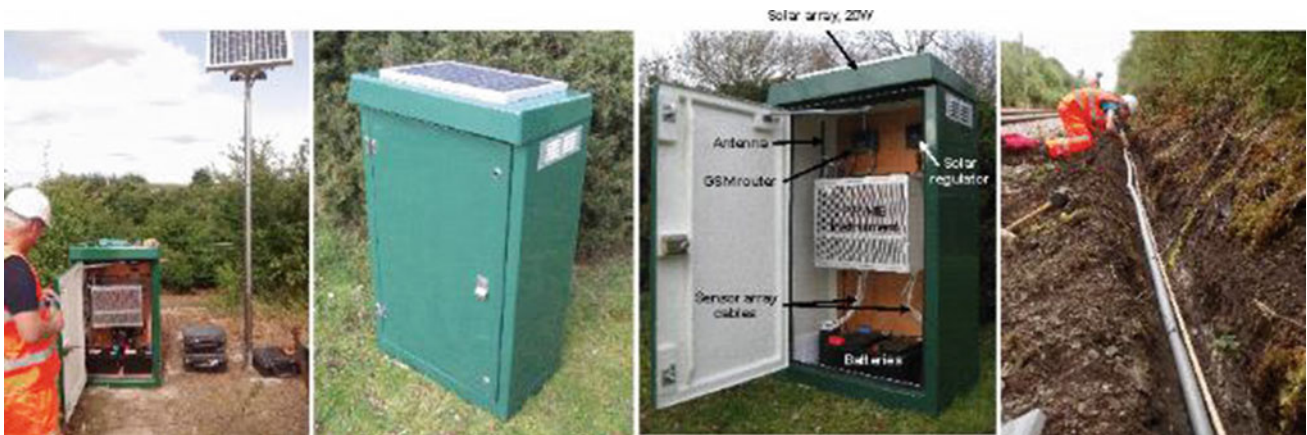
Fig. 2 PRIME system field deployments showing key components and sensor array installation
