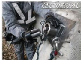
Removal of Wedge
