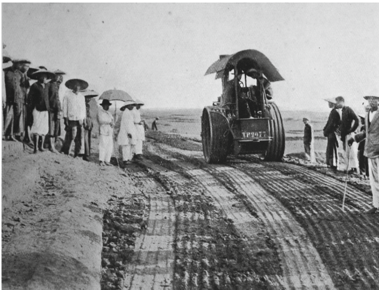
Fig. 7. In the 1930s, for the first time, heavy construction machinery was introduced in Vietnam which had increased the quantity and quality of the dike system in the Red River Delta [5].
