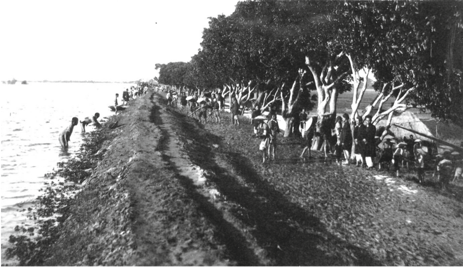
Fig. 4. Pre-colonial dike repair and public works: The mandarins directed the population to repair the dike system and hydraulic works. In the instance above, the work is carried out on a dike in Thai Binh, Red River Delta. [ Source: Dépôt des archives d’outre-mer, Aix-en-Provence: BB/SOM//D3685].
