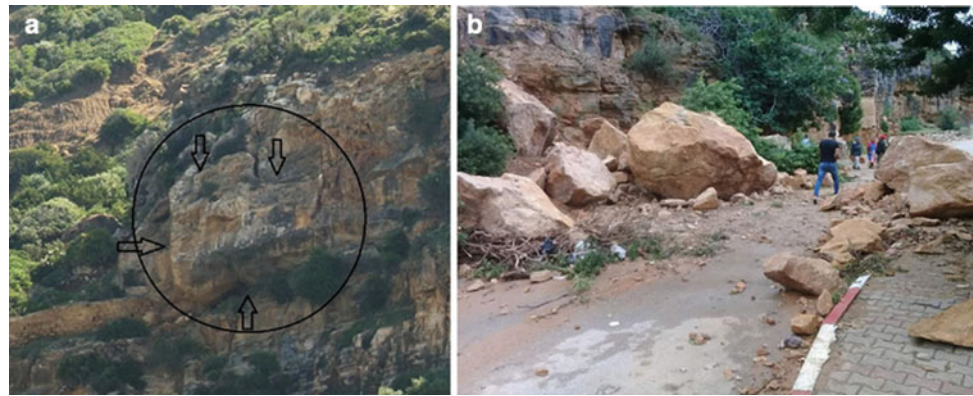
Fig. 25 Example of rockfalls that occurred during heavy rainfall in Korbous, Tunisia. a. Rockfall source that fell down on September 23 rd , 2018, during rainfall reaching 300 mm/2 h. b. Rockfall of blocks on October 17–18, 2018 occurring during a 190 mm precipitation event
