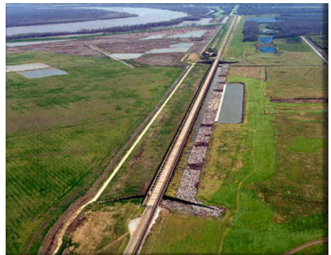
Fig. 18.30 Morganza floodway consisting of a concrete weir equipped with 125 gates to control the flood release. At the land side scouring protection measures are added (photo source:Mississippi River Commission, 2007)
