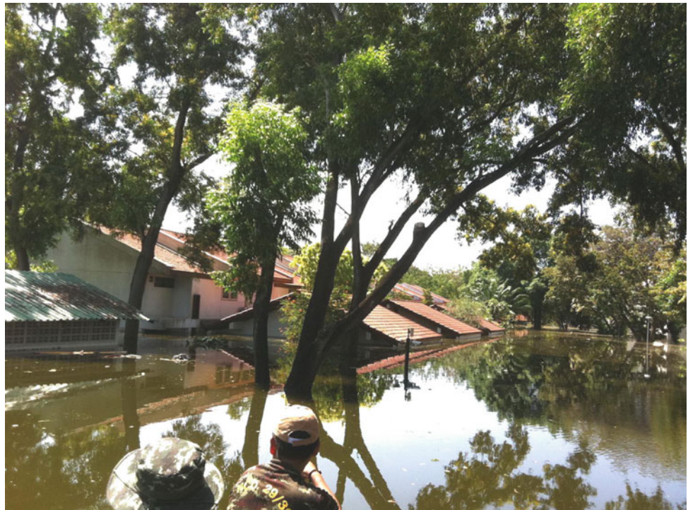
Fig. 22.4 Stagnant ponding flood in a living compound stands for 3 months
