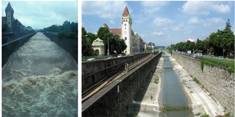
Fig. 18.23 Engineered river profile (city of Vienna): straight and low roughness (a) during a flood event (b) at low flow conditions (Photo source: MA45 Vienna)
