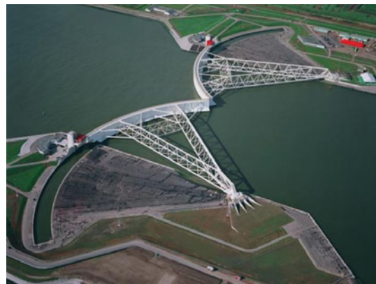
(a) Maeslantkering storm barrier (Riteco, 2017)
