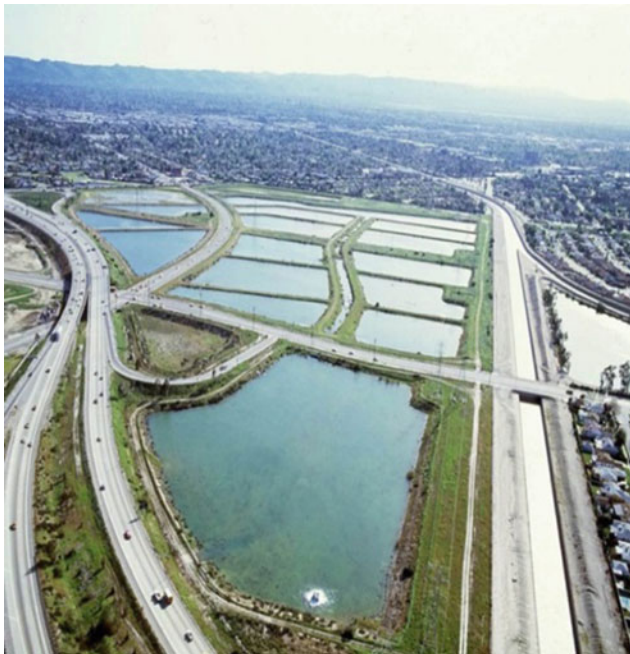
Fig. 23.2 Spreading basin (Source Los Angeles Department of Water and Power www.dpw.lacounty.gov )
