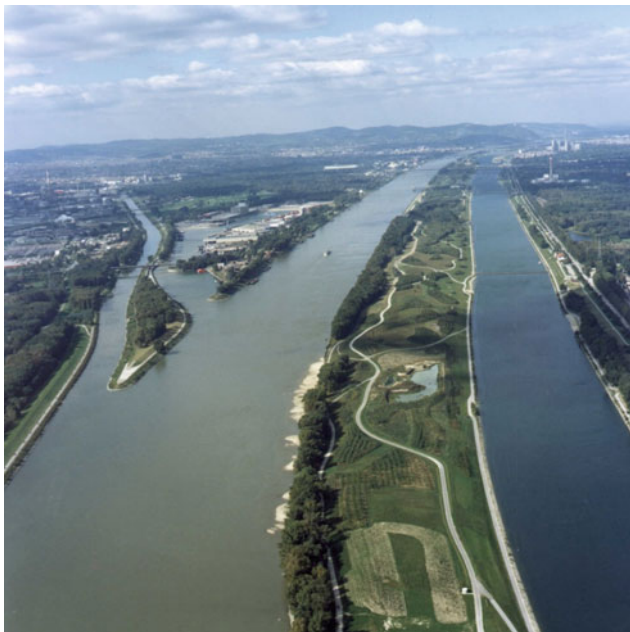
Fig. 18.29 Flood bypass channel in the city of Vienna (before construction of hydropower station Freudenuau) seen from downstream. From left to right: confluence of a side arm (Danube channel), middle: Danube river, Danube island (artificial), and right: flood channel (photo source: Verbund AG, Vienna)
