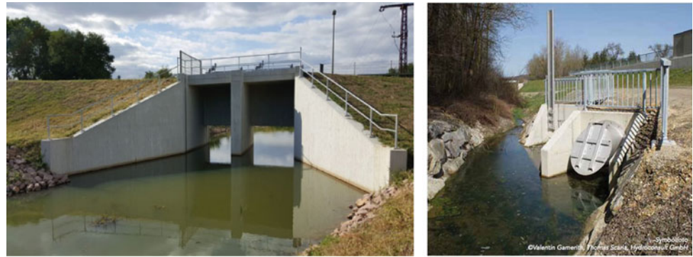
(a) gate controlled culvert
