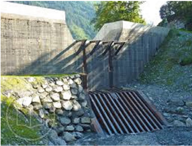
Fig. 18.14 Check dam in headwaters (Anker 2007)
