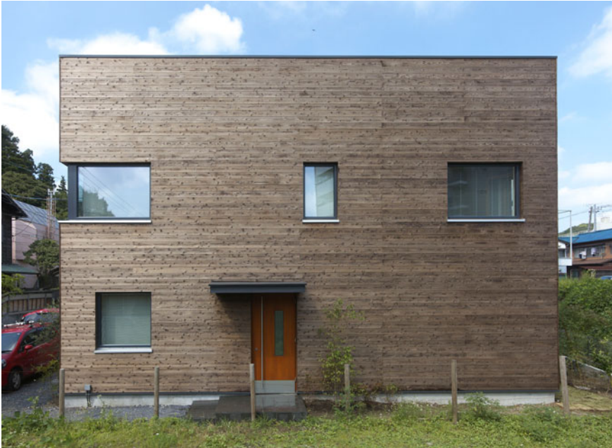
Fig. 12.3 Passive House Kamakura ( Source KEY ARCHITECTS Co., Ltd, reproduced by permission)
