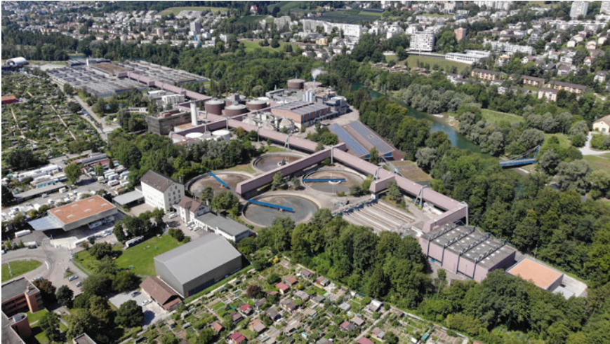
Fig. 12.5 Sewage Treatment Plant Zurich, ERZ Zurich
