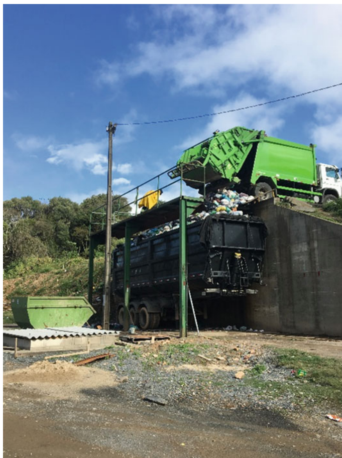
Fig. 7 Image of the transshipment station
