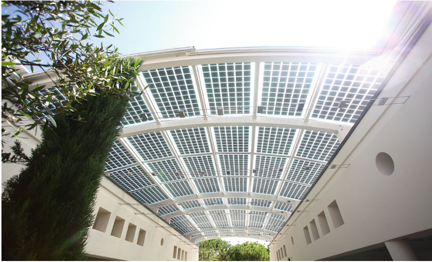
Fig. 9 Photovoltaic system at the Jesolo International Club Camping
