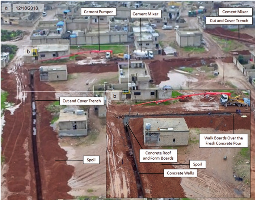
Fig. 14.23 (a) Drone footage released by Turkish media of the YPG/YPJ/SDF held city of Kobane showing construction of CCHTs in December, 2018 (TRTWorld 2018). (b) Higher resolution portion of still frame from ‘a’ shows the concrete walls of the trench and the new section of concrete roof. The new section of roof extends back to the pumper truck and a team is working the concrete pour before laying down boards in preparation for the spoil to be moved to cover the tunnel. Daily Sabah https://twitter.com/DailySabah/status/1075122277589626881
