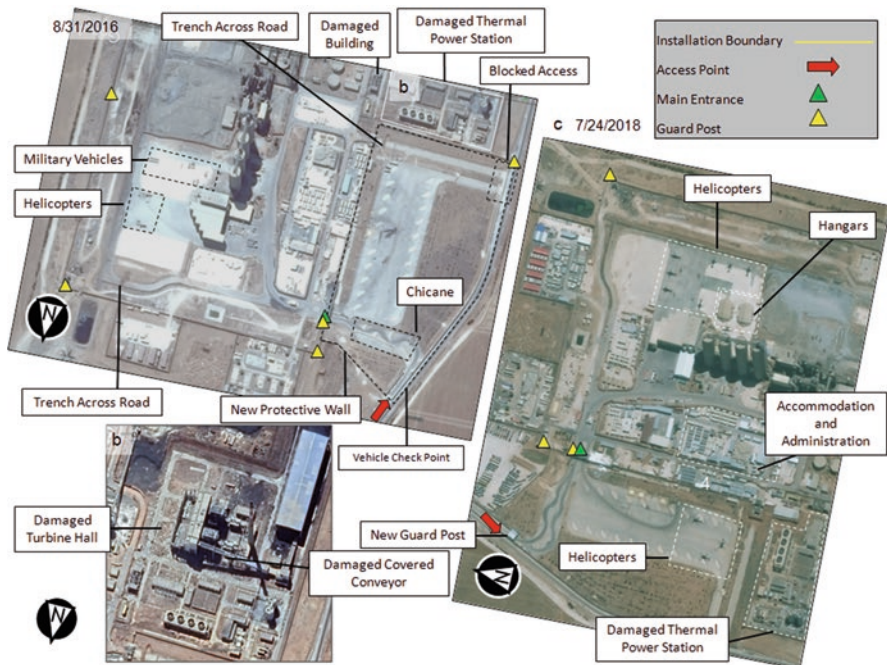
Fig. 14.15 (a) WorldView EO image of the Lafarge Syria Cement Plant acquired on 31 August, 2016 after it was captured from IS by YPG and anti-IS forces. (b) Enlargement of the conventional pulverized coal-fired steam plant showing extensive damage to the two EPs, boilers and turbine hall. (c) WorldView EO image acquired on 24 July, 2018 showing continued use of the LSCF by anti-IS forces. Individual elements within facilities in the plant are identified in (a, b, and c) that were damaged, altered, added or being used for a different purpose
