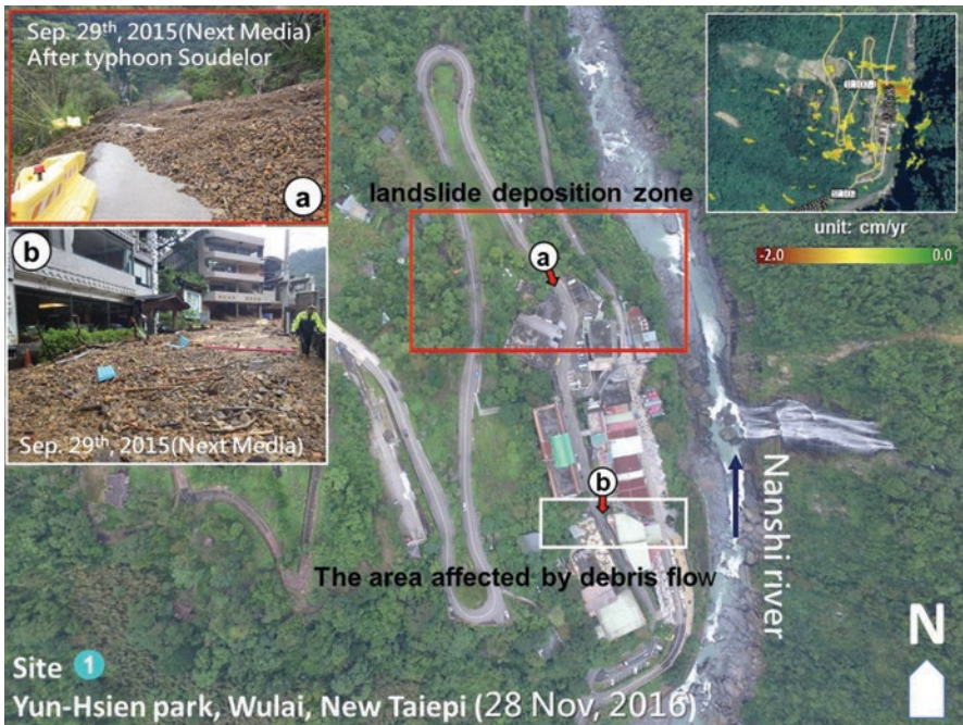
Fig. 5.9 The surface displacement map (LoS) of SBAS and corresponding slope disaster in site 1 (basemap: UAV aerial image)
