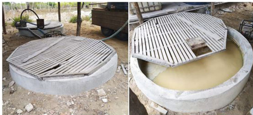
Fig. 1 Cassava wastewater storage tank
