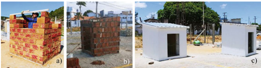
Fig. 8 a T1, earthbag system. b T2, masonry system. c T1 and T2
