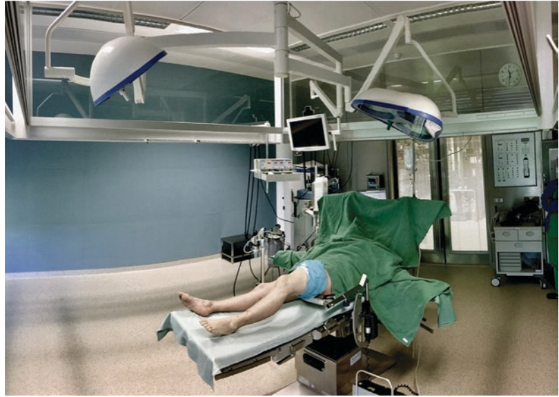
Fig. 20.1 Operating room with laminar air flow ventilation. The patient is positioned at centre of the room
