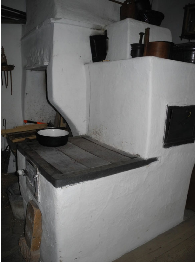
Fig. 6.3 Stoves replaced open fireboxes for meal preparation. They were combined with an oven (on the right) to bake smaller dishes. The bread oven was used for baking bread (in the picture behind the stove on the top left). The method of heating and baking bread remained the same as in the Middle Ages
