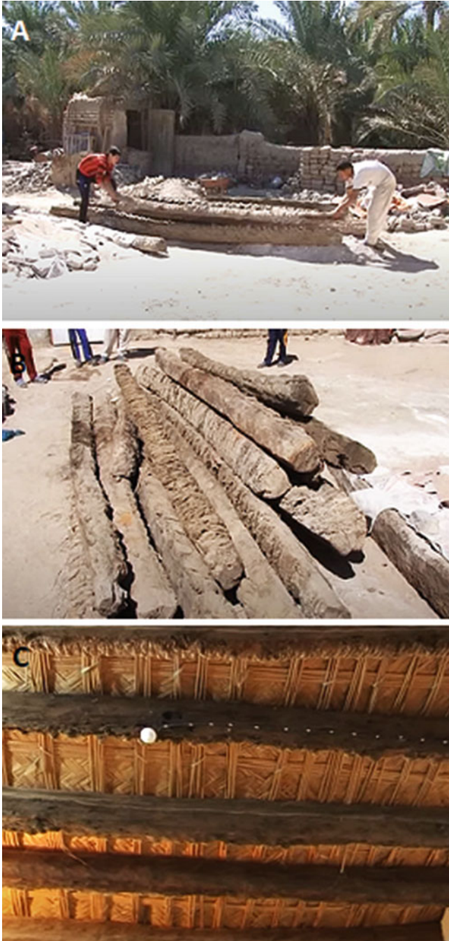
Fig. 28.3 Stems of date palm tree used for house roofing. (a) Date palm trunks prepared for roofing process; (b) date palm trunks after cutting; (c) completed roof
