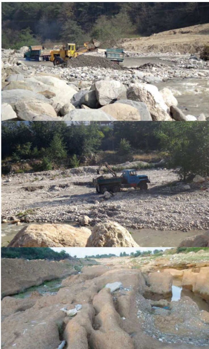
Fig. 52.22 Gravel mining and sand extraction
