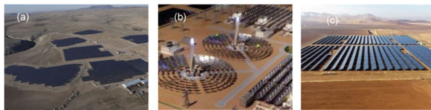
Fig. 14.4 Examples of solar power plans in the ETRB region; (a) Hanwha Q CELLS and Kalyon Enerji win 1 GW solar tender in Turkey; Picture Credit: metecotrol/Phoenix Solar. (b) The Mohammed bin Rashid Al Maktoum Solar Park will have both PV and CSP components, picture credit: Server 2018. (c) Iran’s last major solar power plant in the country’s western province of Hamedan, picture credit: IPTV (2017)
