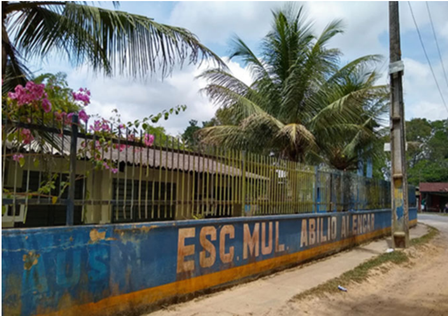
Fig. 1 Facade of Abílio Alencar municipal school
