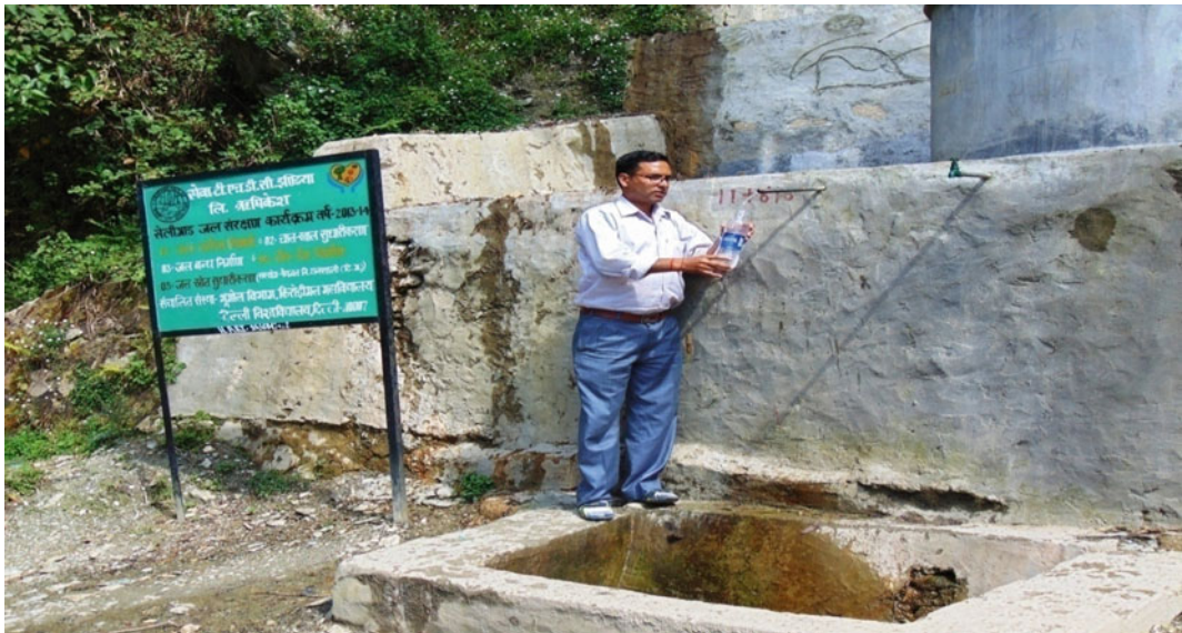
Plate 12.2 Water supply, distribution and management, Dhansali, 2015. Source Primary Survey, 2015
