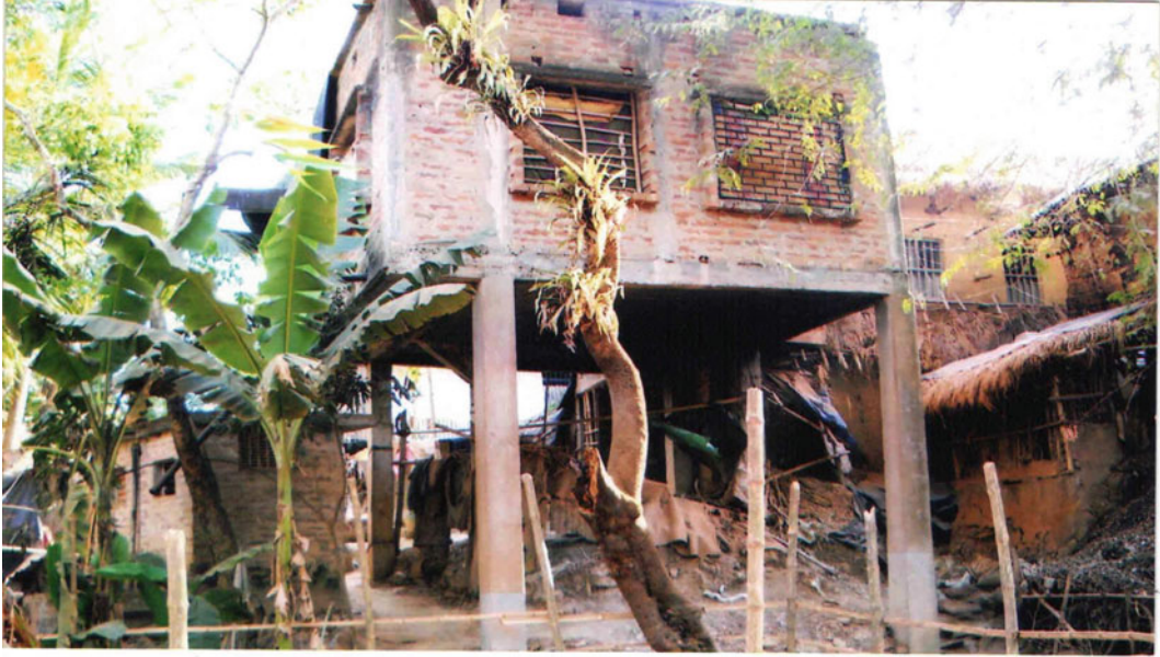
Plate 6.13 Construction of residential building above 15 feet from the ground to reduce the magnitude of damage during the occurrence of flood in Khanakul-II Block
