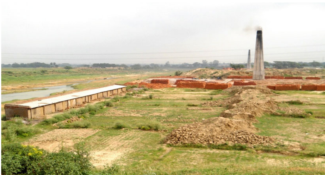
Plate 6.3 Establishment of brick industry in the channel bed of Darakeswar River near Arambagh, a clear evidence of encroachment, which obstructs the natural flow and increases the chances of flood during the period of heavy rainfall
