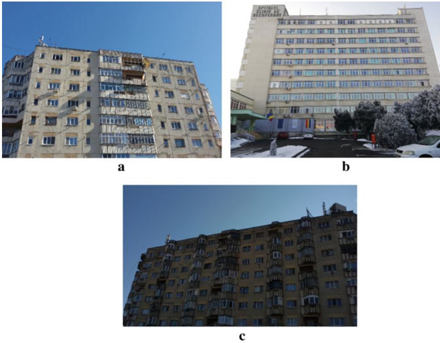
Fig. 1.21 a Blocks of flats b Hospital c Blocks of flats in need of deep retrofit in Romania
