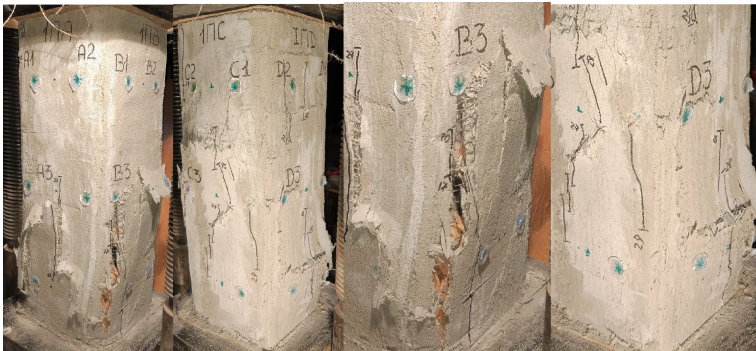
Fig. 6. Failure mode and appearance of strengthened specimens
