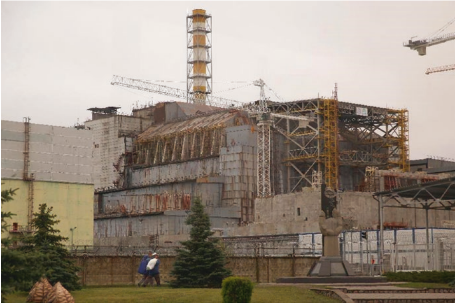
Fig. 29.7 Encasement of Chernobyl nuclear power station, Ukraine
