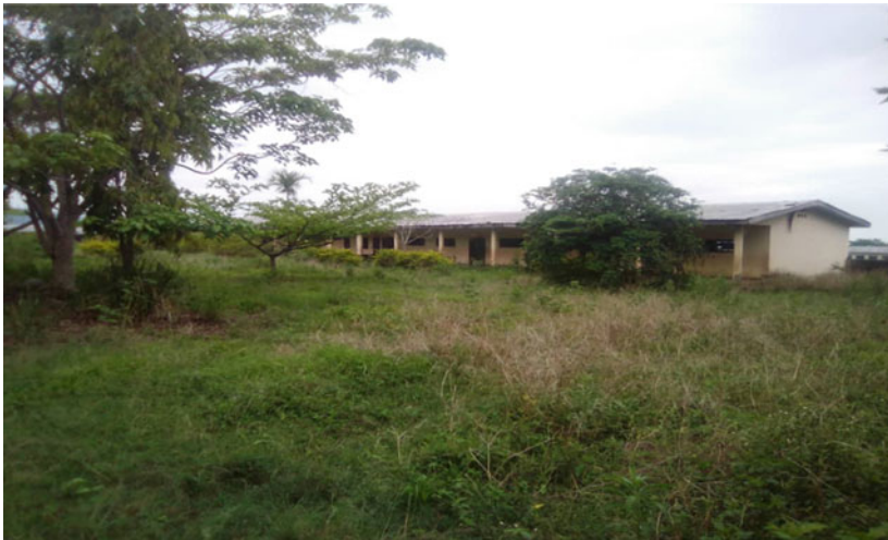
Fig. 3.4 An abandoned school site due to armed conflict (February, 2020)
